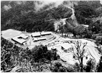
The Yadana Project's facilities on the Thai-Burma border.
