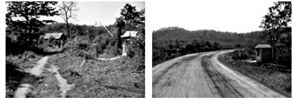
“Before” and “after” pictures of the Zinba road from Total’s website.
