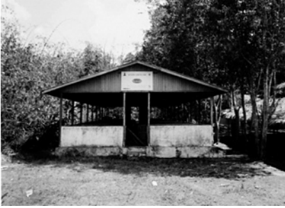
The abandoned pig farm in Michaunglaung. The sign on the building displays the Yadana Project logo.
